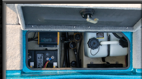
Very easy access to chargers, batteries, oil, and pump through the rear hatch.
